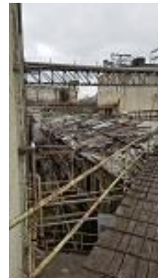
Mill J roof
