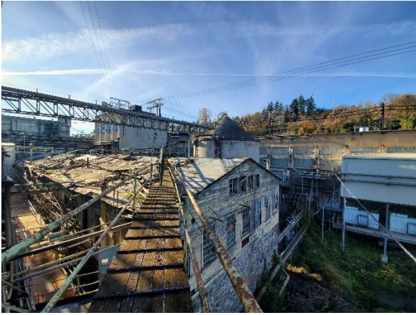
Mill J before demolition
