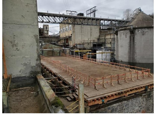
Mill J foundation after demolition
