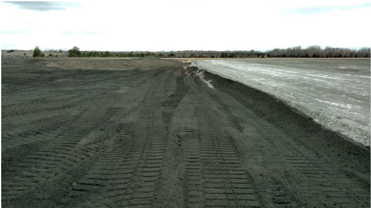
Completed grading of bottom ash to form slope westward to stormwater retention area over previous ditch between bottom and fly/economizer ash
