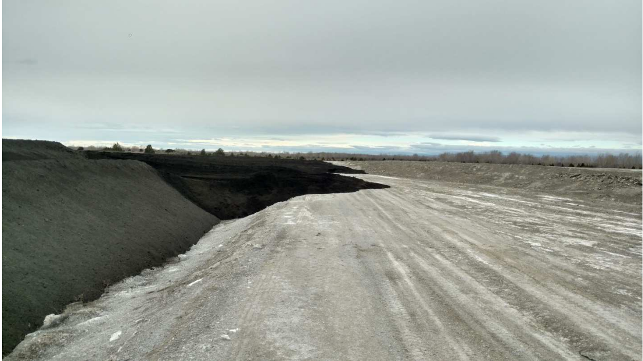
Bottom ash being graded north over large ditch between bottom and fly/economizer ash piles.
