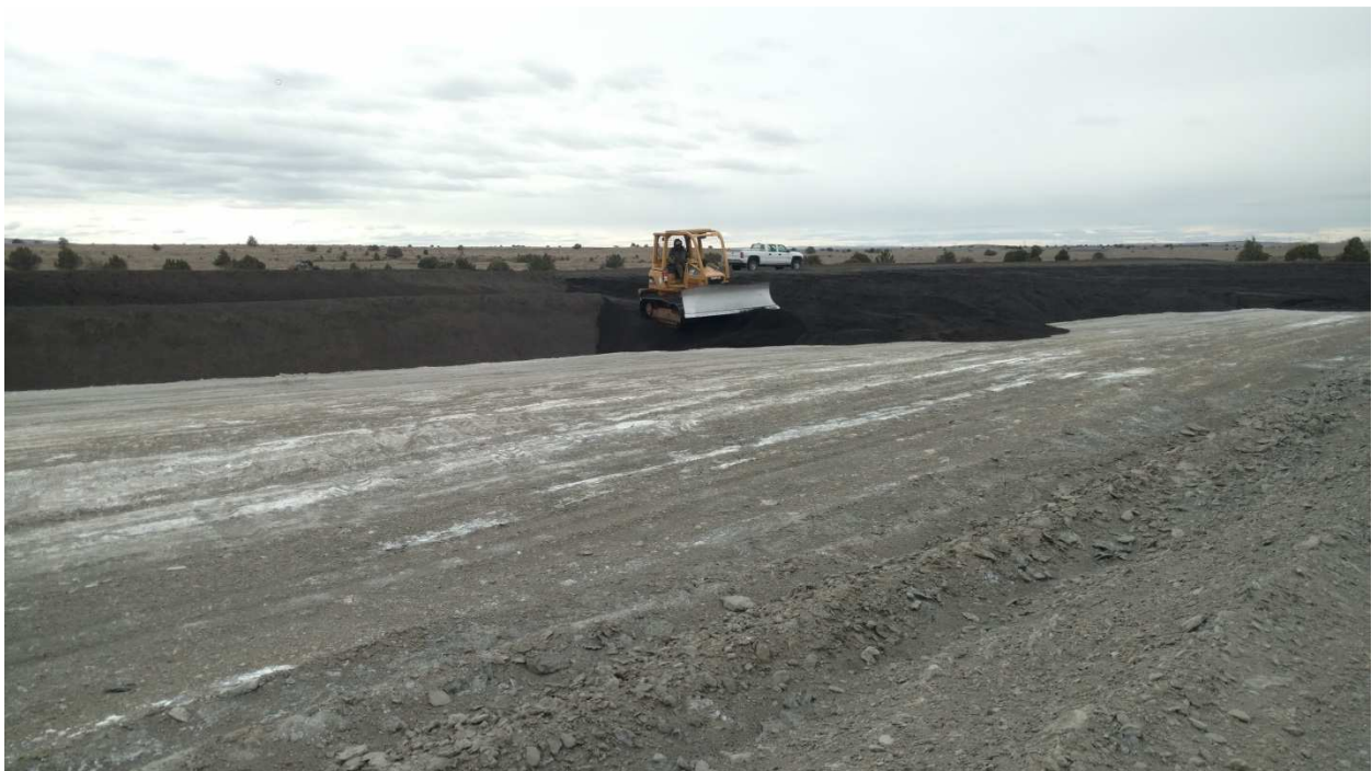
Small dozer used for grading bottom ash toward fly/economizer ash.
